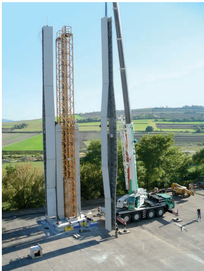
Fig. 14. The large-scale test structure during erection
