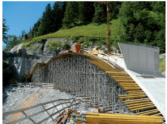
Fig. 1. Falsework for the arch of the Egg-Graben Bridge
