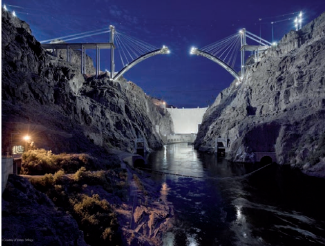
Fig. 3. Hoover Dam Bypass (photo credit: Jamey Stillings Photography, USA)
