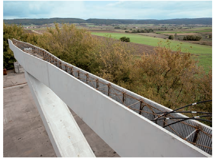
Fig. 18. Bridge girder with 70 mm prefabricated wall elements
