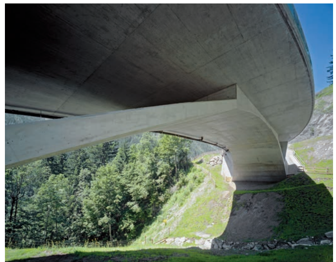
Fig. 2. Egg-Graben Bridge (photo credit: Pez Hejduk, Austria)
